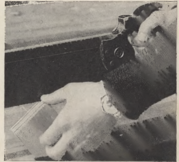
Fig. 195. Sawing cheek cuts of tenon
